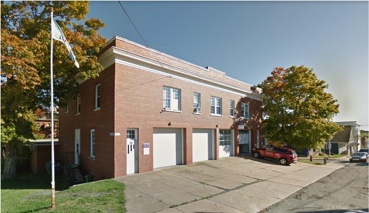
Old Fire Hall Building facing Duke Street
