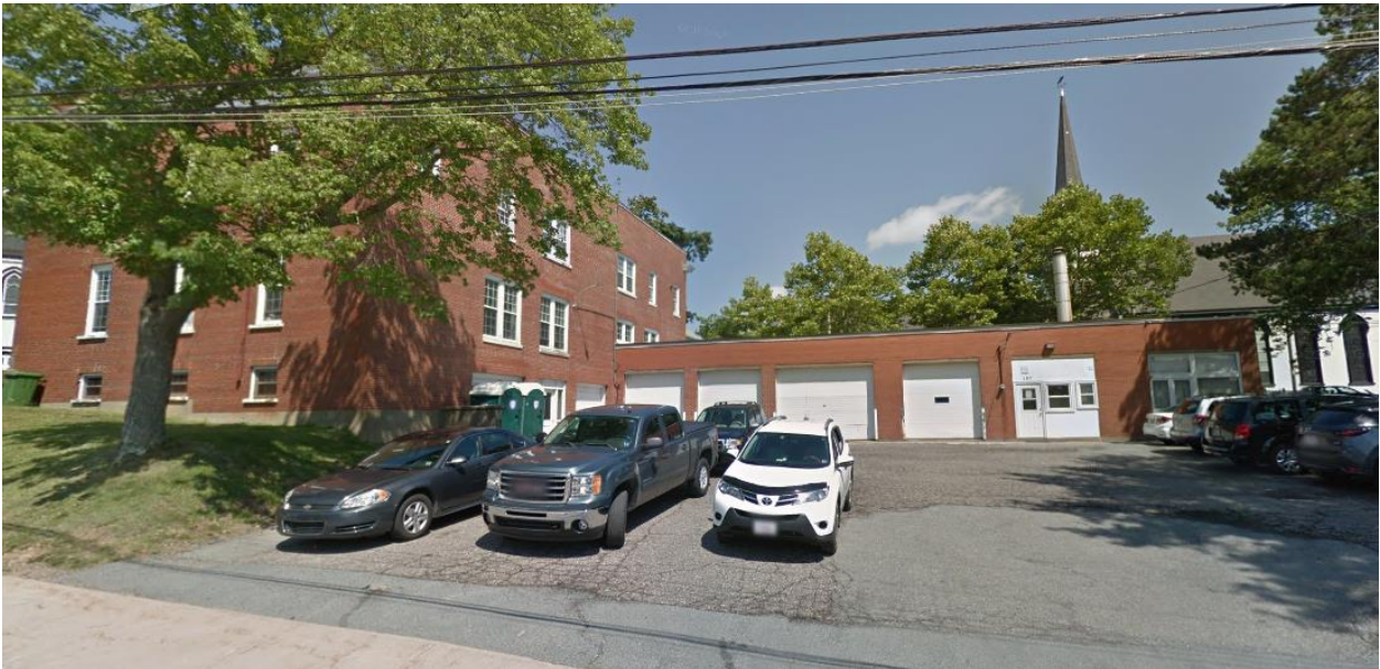
Electric Utility Building Facing Cumberland Street
